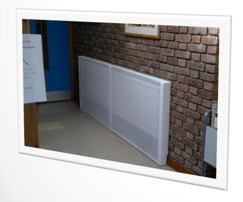
VARIAPLAN Free Flow Pipe Covers are available in 'matching' perforated steel and are designed to complete the installation and allow the pipes to provide maximum 'useful' heating output
